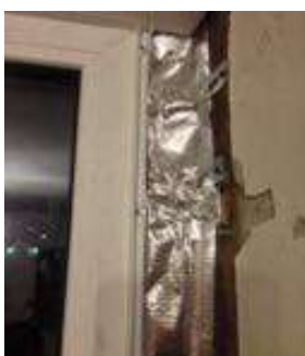
Pictures 7 and 8. Vapour seal tape (foiled tape, left) and installation wedges, fixed with foam (right)
