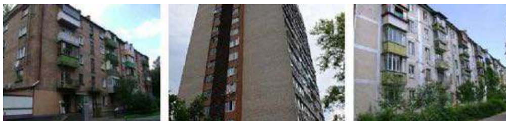
Figure 12: 480-series: left: 5-storey brick building, middle: 16- storey brick building, right: modification of reinforced concrete panels [31]
