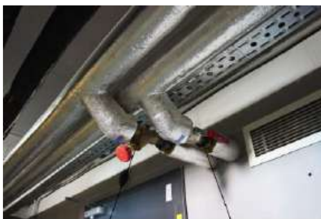
Balancing valve on return riser Shut-off valve on supply riser
