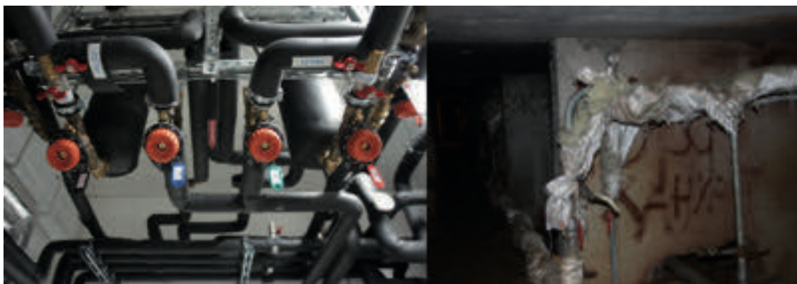
Figure 10. Insulated pipes and non-insulated pipes
