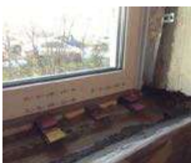
Pictures 7 and 8. Vapour seal tape (foiled tape, left) and installation wedges, fixed with foam (right)
