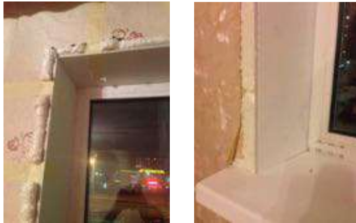
Picture10. Installation foam (left), vapour seal (right)
