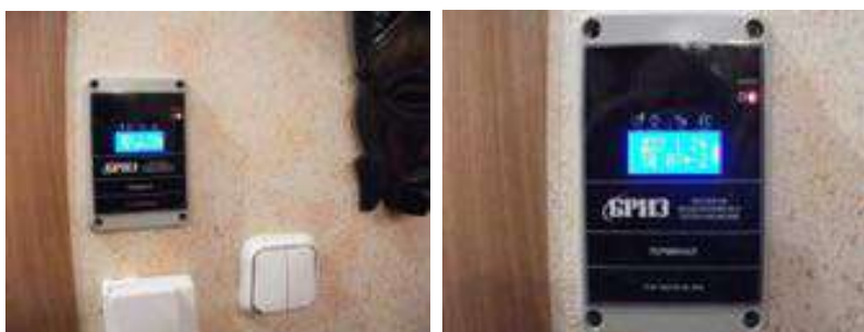
Figure 15. Automatic regulator of air exchange and flat heating.
