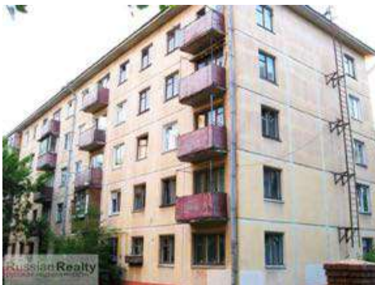
Figure 8: Series 1-335, widely spread in Russia, Belarus and Ukraine – are lightweight five-storey buildings with an insulation layer of mineral wool on the exterior walls and interior partitions with a thickness of a few centimeters. They are characterized by large heat losses and low sound insulation. Due to these main drawbacks, houses of series 1-335 are to be demolished in Moscow from 2015-2017. In St. Petersburg, houses of series 1-335 are subject to refurbishment; some quarters are scheduled for demolition as well. [3]
