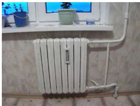
Figure 21. Heat cost allocator installed on heating device
