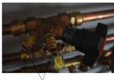
Connections for pressure drop measurements
