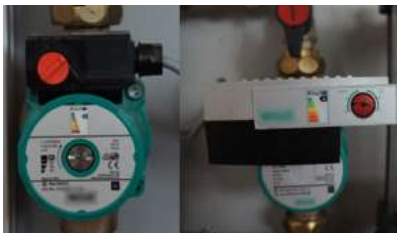
Figure 12. Example of circulation pumps with different efficiency classes.
