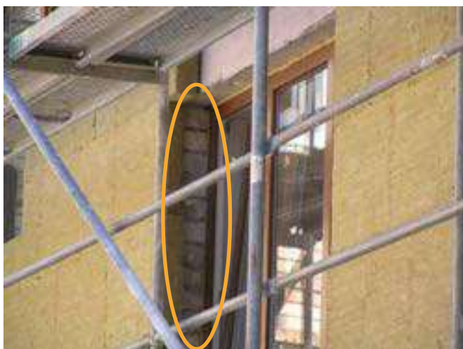
Figure 9. The yellow ellipse shows a potential thermal bridge. Further insulation is required to eliminate it.
