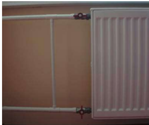
Figure 7. Panel radiator connection to existing single pipe system with bypass and shut-off valve
