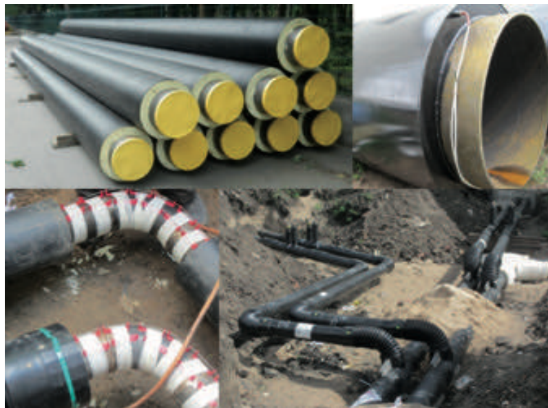
Figure 2. Modern pre-insulated pipes for district heating systems
