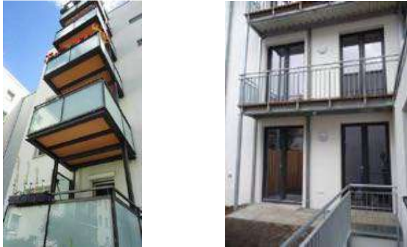
Figure 13. Balconies with own load-bearing structure, separate from building envelope
