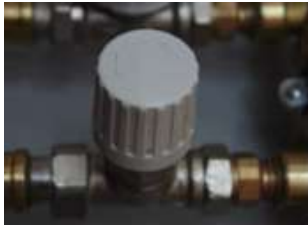
Figure 14. Valve for manual setting of water flow
