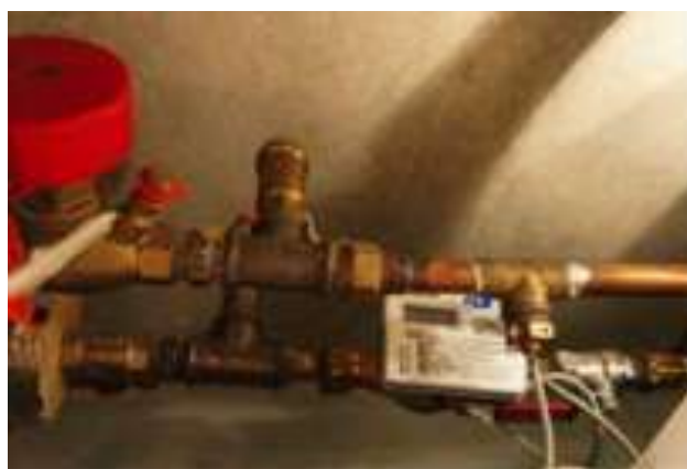
Figure 21. Practical installation of direct heat meter
