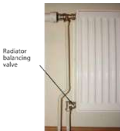
Figure 19. Balancing of heating elements
