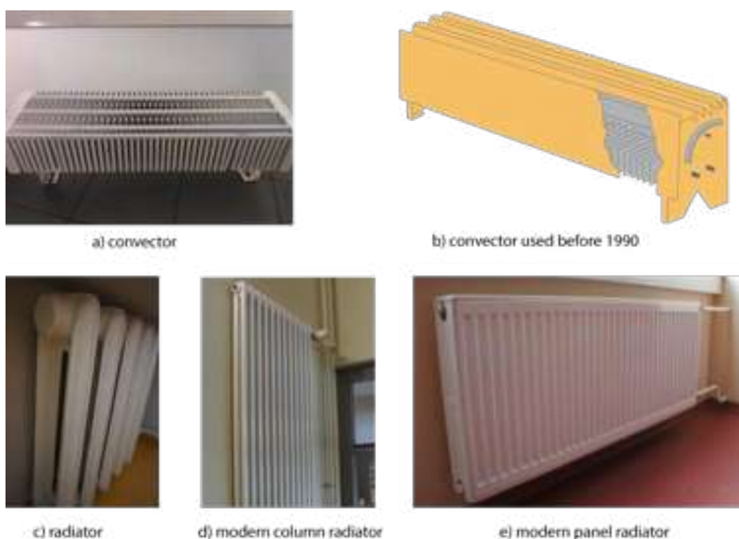
Figure 3. Heating elements: a) convector b) convector used before 1990 c) radiator d) modern column radiator e) modern panel radiator
