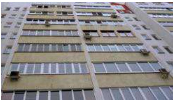
Figure 13. Boxes of air conditioners on facades of residential buildings can be a first indicator that overheating in summertime is an issue.
